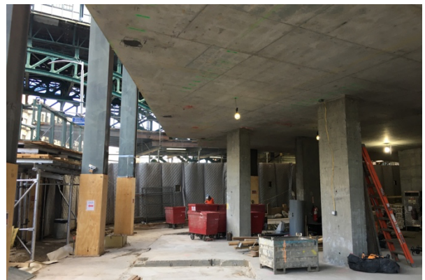
Ground floor of 600 W. 125th Street, looking east
