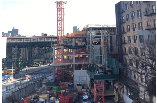
600 W. 125th Street, looking east
